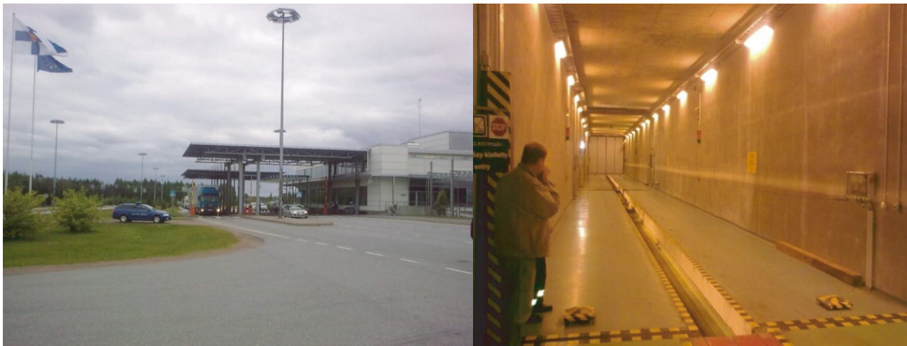
FIGURE 24. PURPOSE-BUILT X-RAY AT VAALIMAA AND BCP INFRASTRUCTURE
